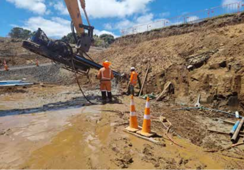
Ground anchor tests underway for the new retaining wall.
