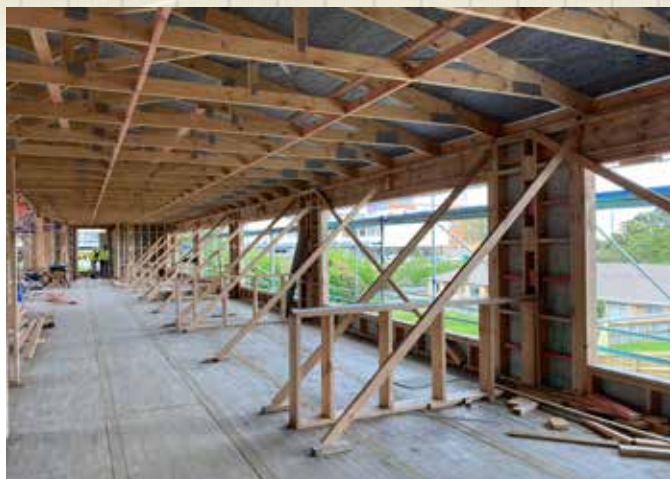
Timber framing has been completed and the internal fitout is underway.
