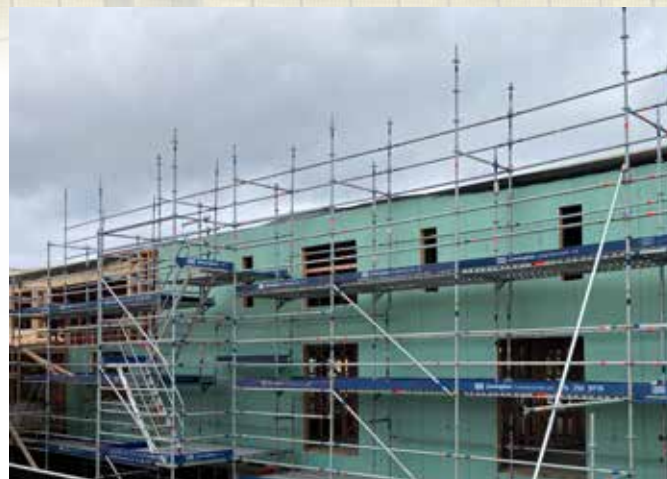
External linings and roof installation underway.
