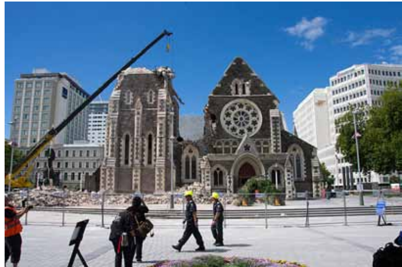
■ Christchurch Cathedral after the February 2011 earthquake
